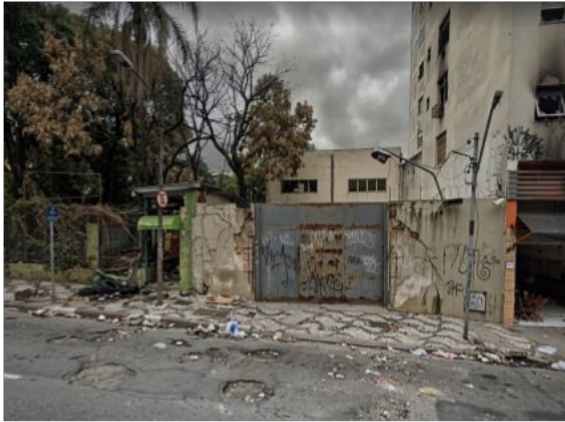
make it unsafe
