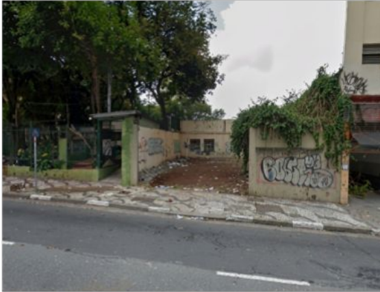
make it unsafe
